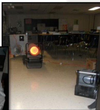
Heating & ventilating impacted space to remove fugitive mercury vapor.
