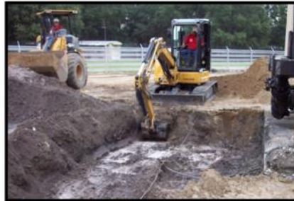
A-C-T excavating MODEF bearing soils.
