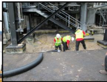
A-C-T excavating impacted soils with vacuum truck.
