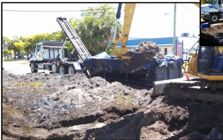
A-C-T personnel excavating impacted soils.
