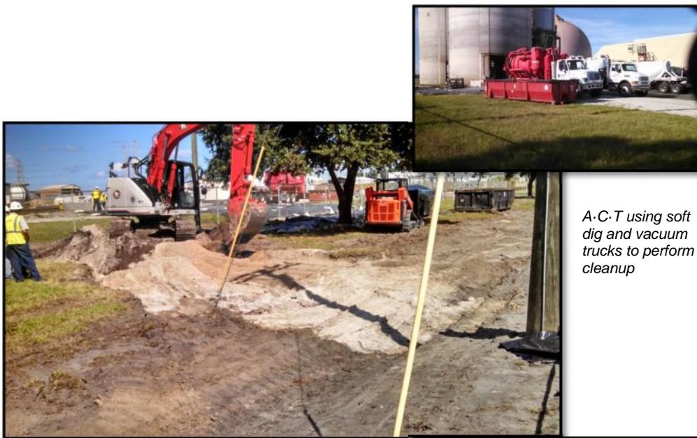
A-C-T personnel excavating impacted soils.
