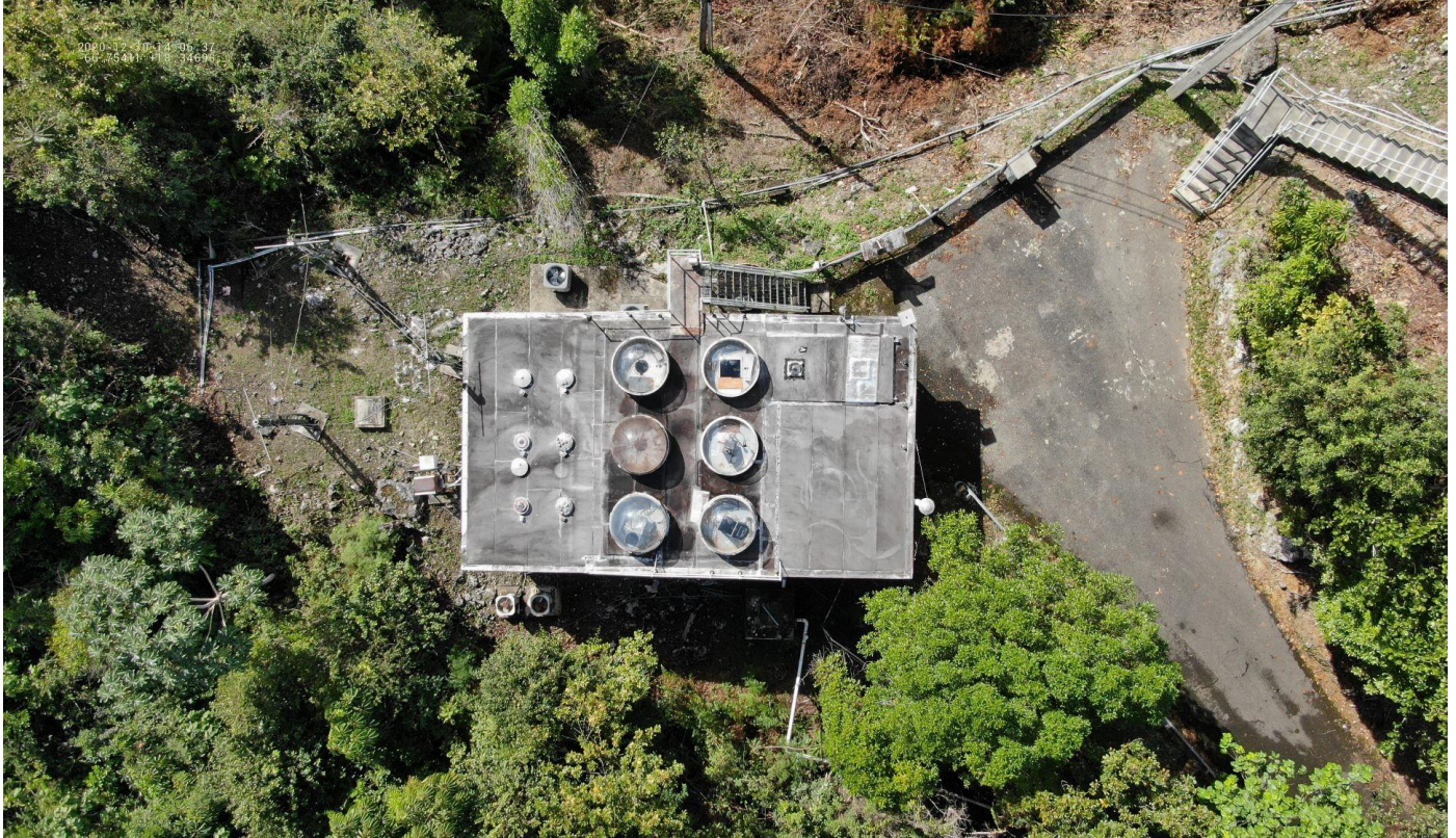
Optical Lab (Aerial View)
