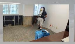
United Restoration performing HEPA vacuuming on mold affected drywall in a local government building after Hurricane Irma.
