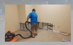
United Restoration maintaining a clean workspace after executing an emergency dry-out and removing water damaged drywall.
