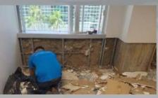
United Restoration removing water damaged drywall in a local government building after Hurricane Irma.
