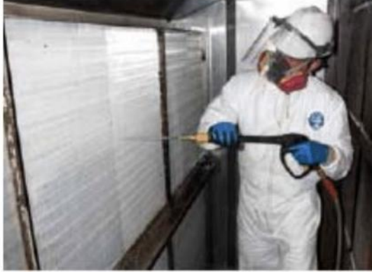
Professional Chill Water Coil Cleaning
