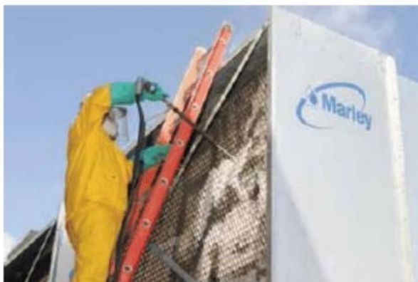
Cooling Tower Fill Cleaning
