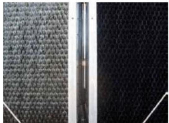
Cooling Tower Fill: Before and After Cleaning
