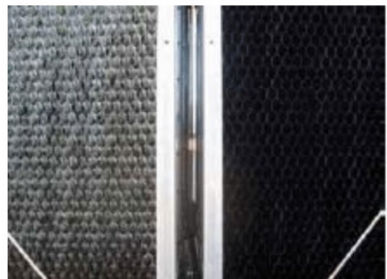
Cooling Tower Fill: Before and After Cleaning
