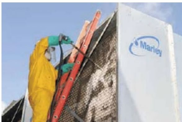
Cooling Tower Fill Cleaning
